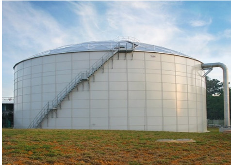
Rolled, Tapered Panel Bolted Tank
